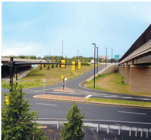
Construction Engineering, Administration and Inspection for Route 18 Extension / Rutgers Improvements - NJDOT 2006 ACEC Patinum Award Winner
